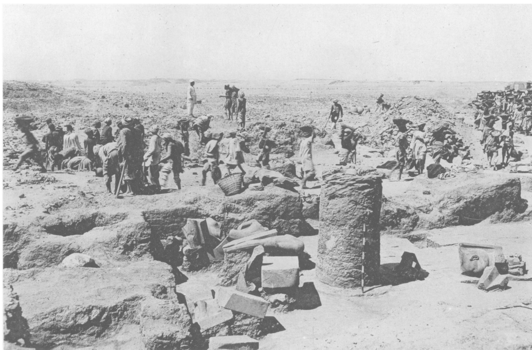
Room B904, seen from the "south-west" corner, with fragments of statues in situ
