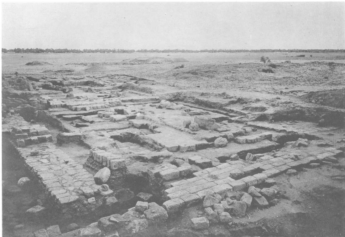
B800, from the "south-east" corner, looking towards the river
